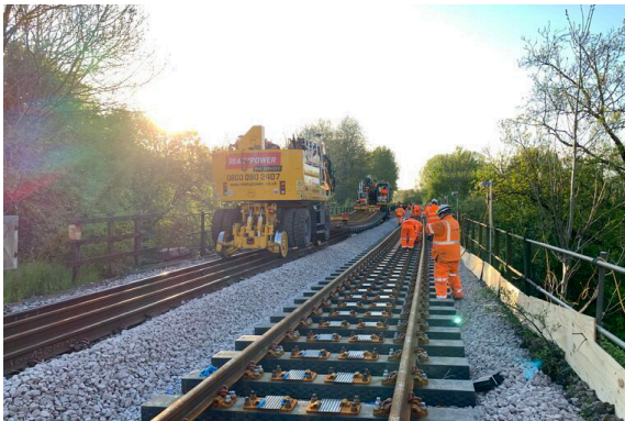
Sicut sleepers being installed on Sherrington Viaduct
