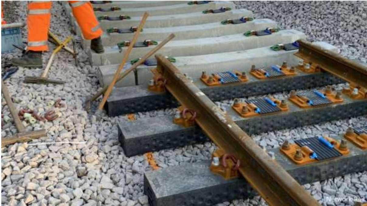
Composite sleepers and the concrete ones they replaced.
